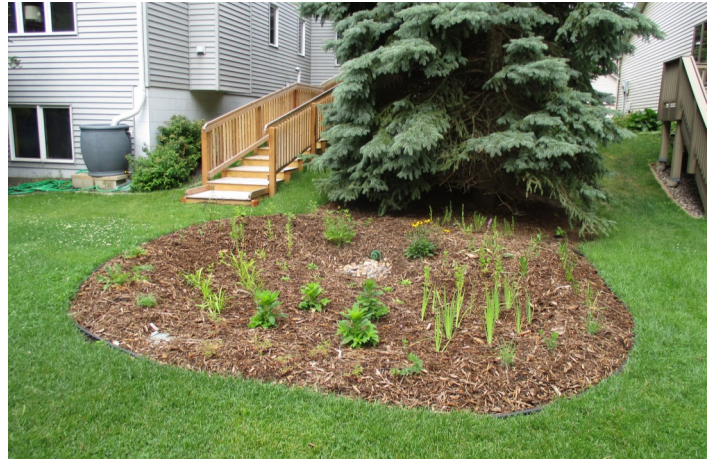
A newly installed raingarden within the Watershed is already capturing runoff and filtering pollutants. Soon the native plants will grow and provide a beautiful landscape amenity.
